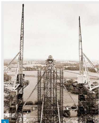
Photo 1: The success of the 218ft fixed transit antenna underpinned the ambition to build a fully steerable paraboloid of similar aperture. (Glyn Evans) Photo 2: The 27ft diameter gun turret rack (left) and trunnion assembly with large roller bearing (right) were hoisted in 1955. (Jodrell Bank) Photo 3: The two cranes have just hoisted the trunnion bearing to the northern tower. (Jodrell Bank) Photo 4: The beginnings of the paraboloid are apparent as the ribs are mounted. For scale, note the two men working on the right side outer connecting panel. (Jodrell Bank) Photo 5: During construction the skeleton bowl was supported by 90 miles of scaffold tubing. (Jodrell Bank)
